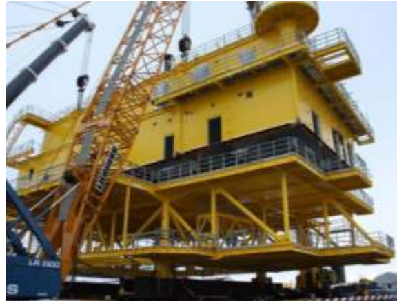
Steel structures fabrication GSG, EPG, MPG
